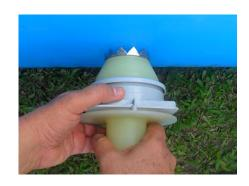
Holding the valve by the frame, twist the hole punch clockwise to firmly tighten the nut.
